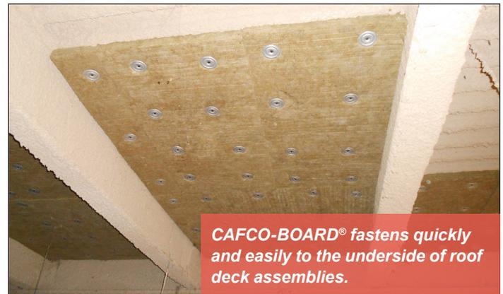
*CAFCO-BOARD<sup>®</sup> fastens quickly and easily to the underside of roof deck assemblies.*
