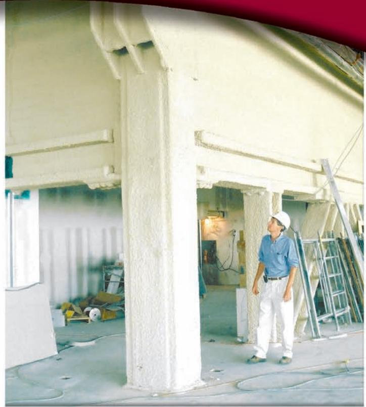
CAFCO-BOARD is a UL classified rigid, mineral wool board that provides up to 4 hours fire protection for columns and up to 3 hours fire protection for beams. CAFCO-BOARD is mechanically fastened to structural steel and is ideally suited for high-traffic and limited clearance areas. CAFCO-BOARD possesses a worldwide reputation for being an exceptional performer in both the Commercial and Industrial sectors for the fire protection of structural steel.
